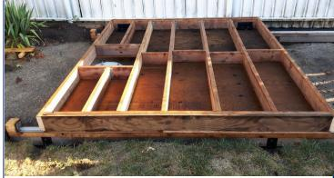
wood joists are used on the sides to distribute the weight to the wheel.
