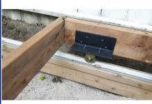
angle-bracket welded onto flat-bar to prevent warpage. Although more expensive, I selected stainless steel since coldrolled steel would rust and aluminum would pit when sand or gravel were on the track.
